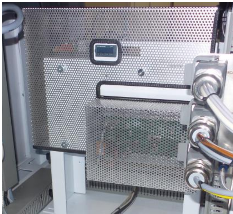
Figure 9: Installing control unit's protective cover
